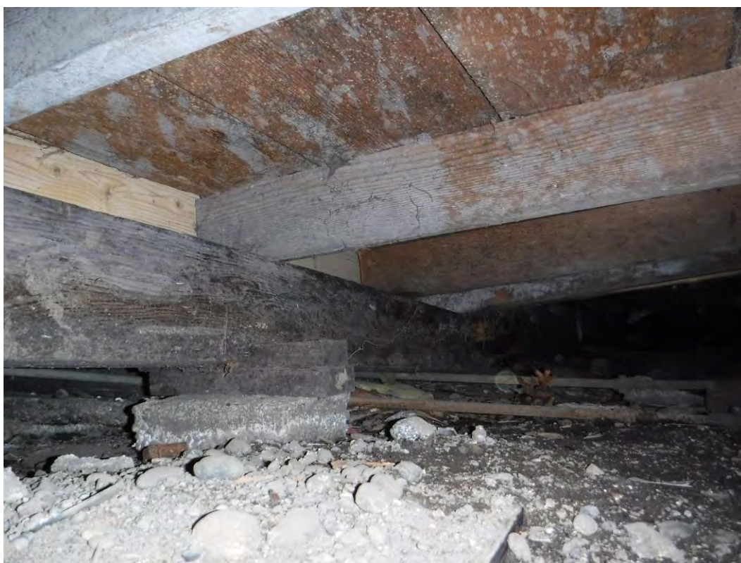
Photograph 15: Underside of first floor.
