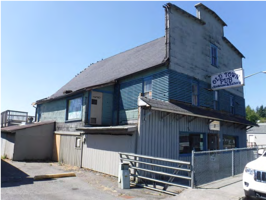
Photograph 6: Northeastern exterior corner of building.
