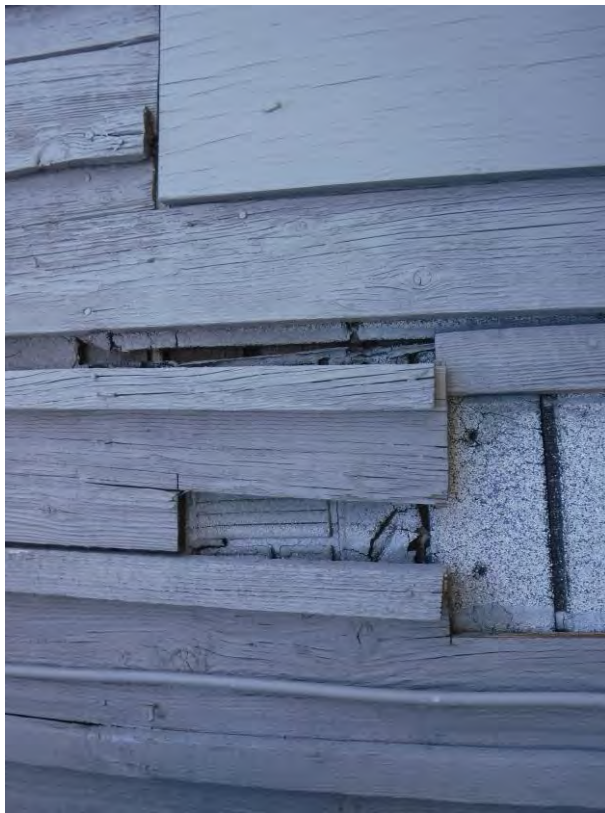
Photograph 7: Typical exterior shiplap.
