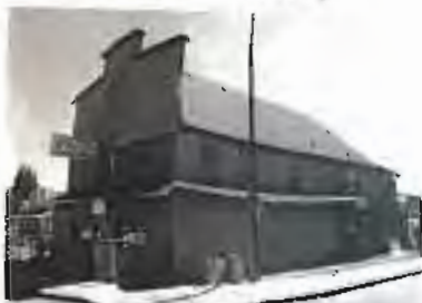
Photograph 2 Another exterior view of building
