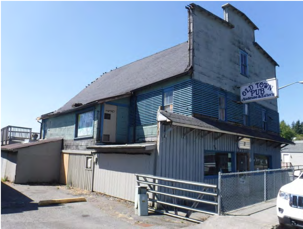
Photograph 6: Northeastern exterior corner of building.
