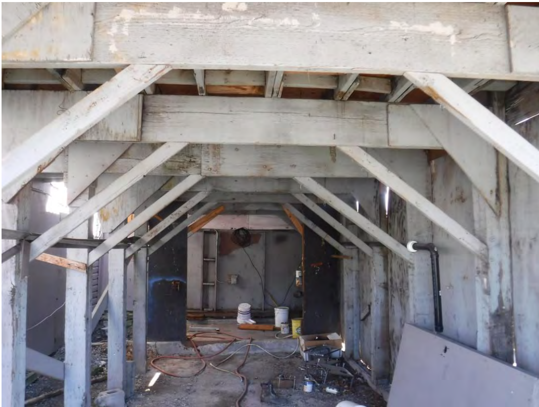
Photograph 8: Underside of deck at southern side of building.
