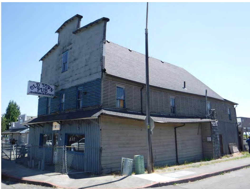
Photograph 2: Northwestern exterior corner of building.
