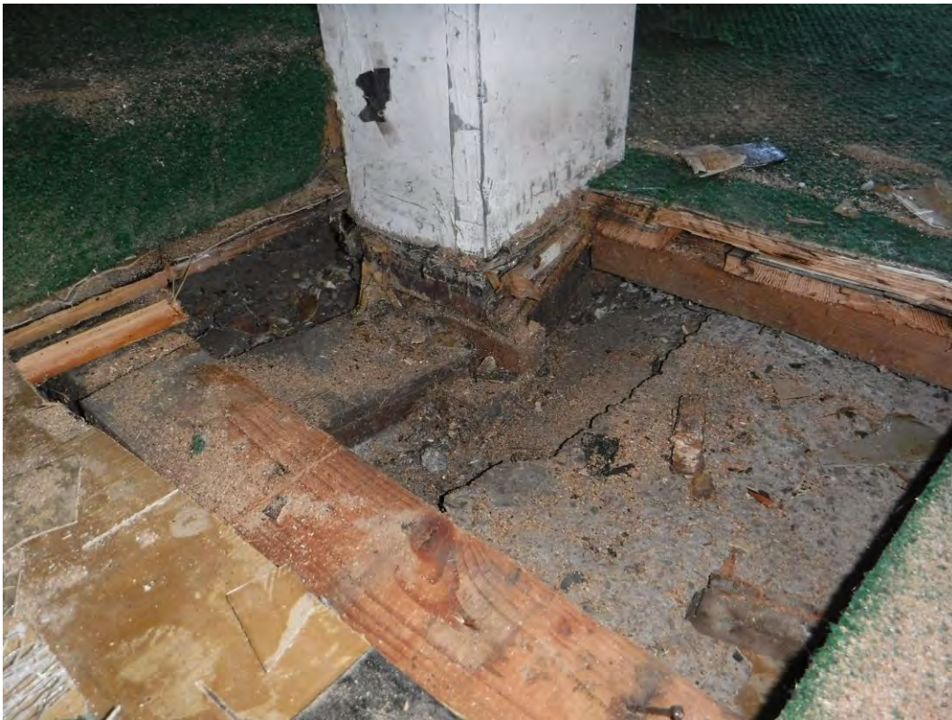
Photograph 10: Hole cut at column base at first floor.
