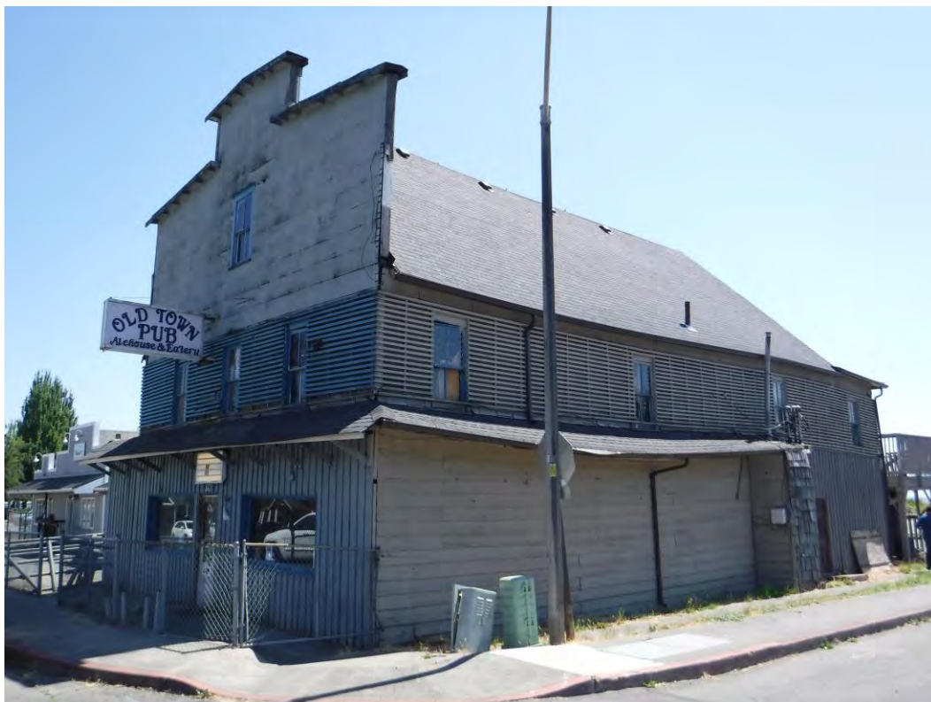
Photograph 2: Northwestern exterior corner of building.
