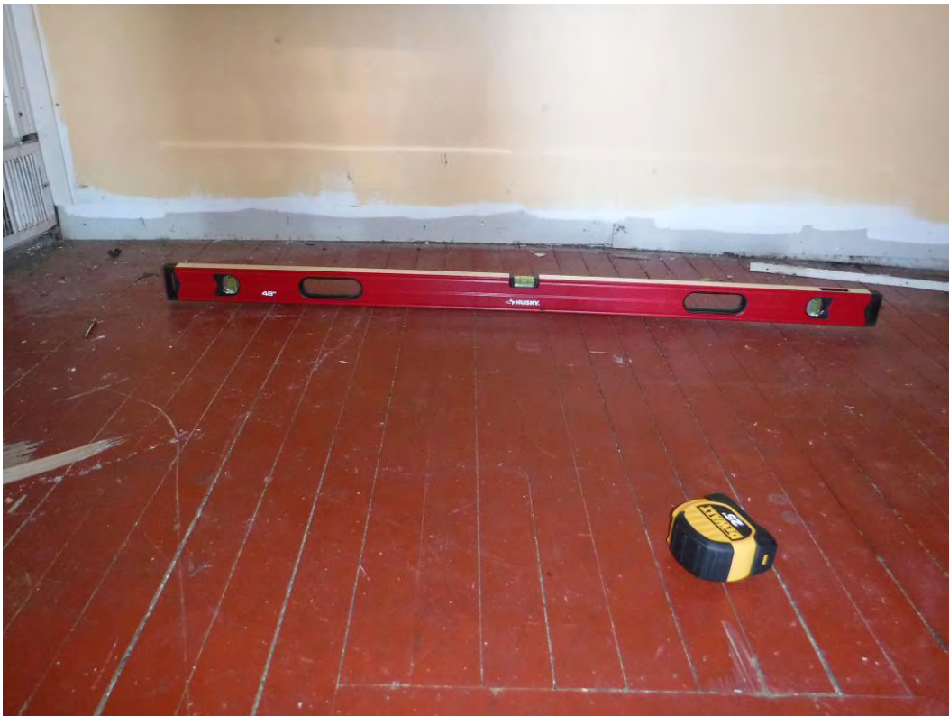
Photograph 12: Second floor at building center with high point (slope east and west).
