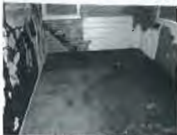
Photograph 4 Interior view of building showing concrete floor
