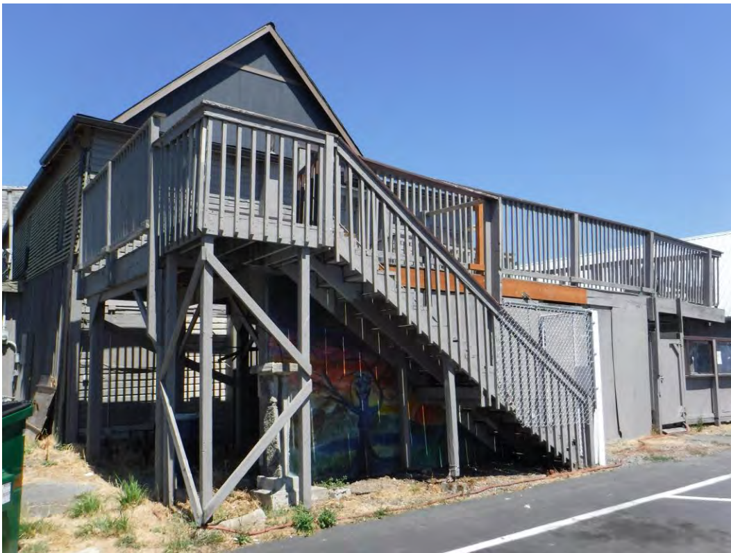
Photograph 4: Deck at southern exterior of building.
