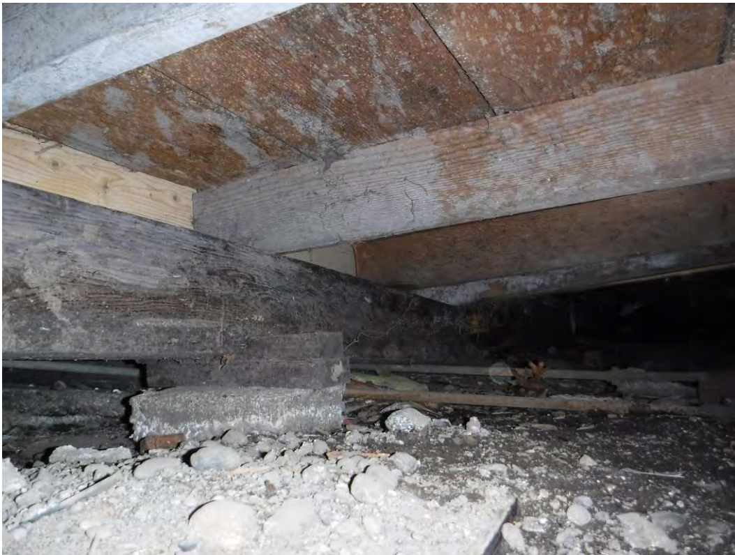
Photograph 15: Underside of first floor.
