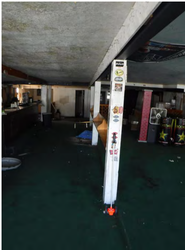
Photograph 9: Interior line of columns at first floor.
