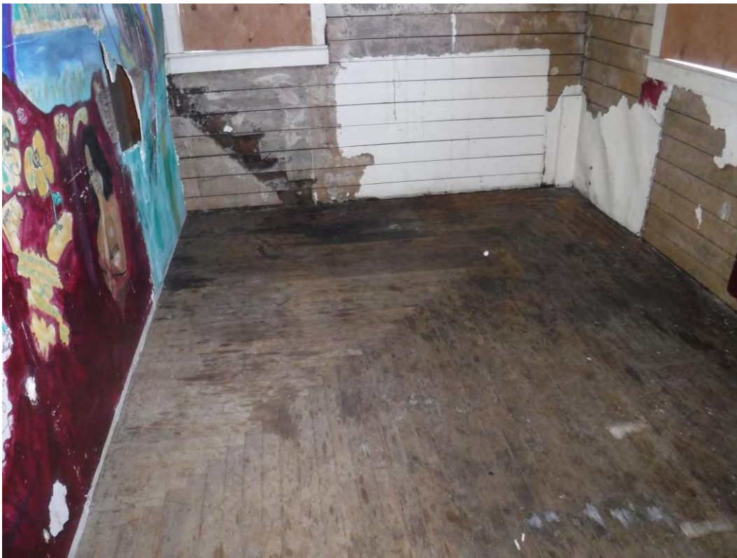
Photograph 11: Typical floor and walls (second floor shown).
