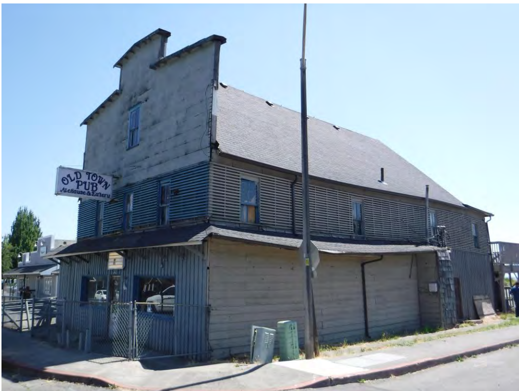
Photograph 2: Northwestern exterior corner of building.
