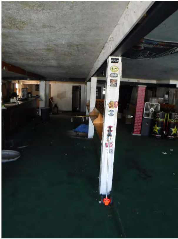
Photograph 9: Interior line of columns at first floor.
