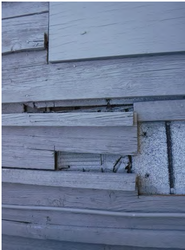
Photograph 7: Typical exterior shiplap.
