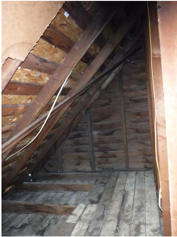
Photograph 14: Western interior with exposed truss top and bottom chords.
