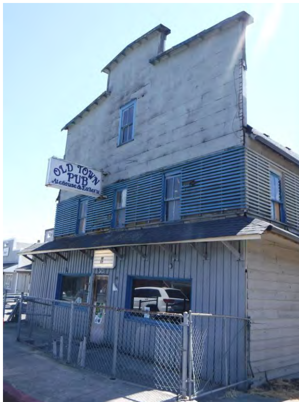
Photograph 1: Northern exterior of building.
