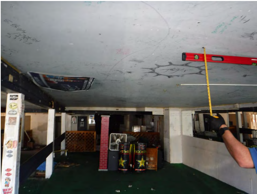
Photograph 11: Underside of second floor with slope toward exterior of 12-inch per 1-foot.
