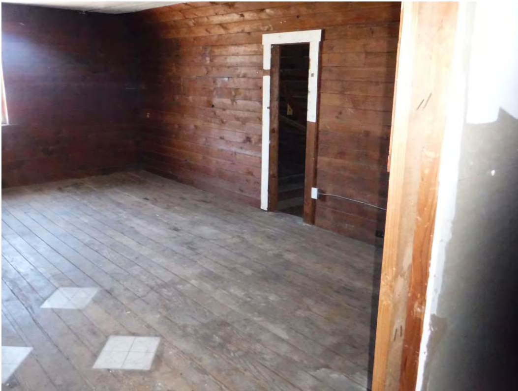
Photograph 13: Typical floor and walls (third floor shown).
