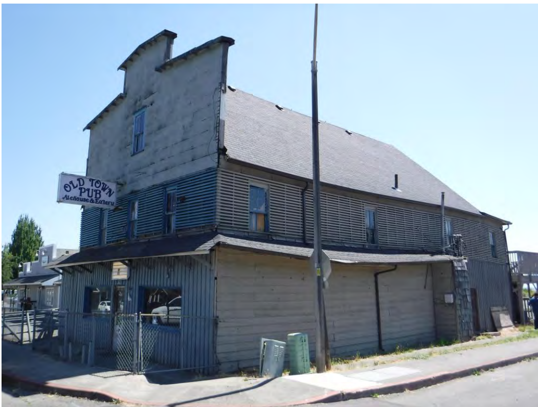
Photograph 2: Northwestern exterior corner of building.
