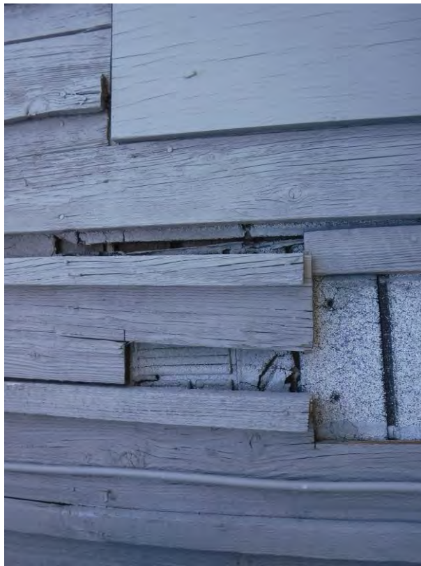
Photograph 7: Typical exterior shiplap.
