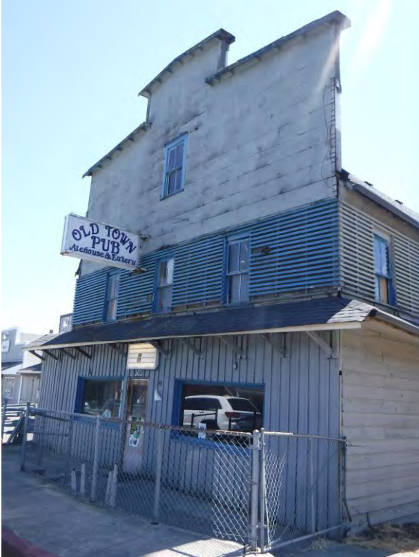
Photograph 1: Northern exterior of building.
