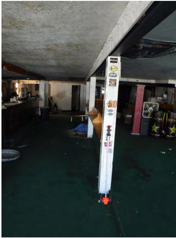
Photograph 9: Interior line of columns at first floor.
