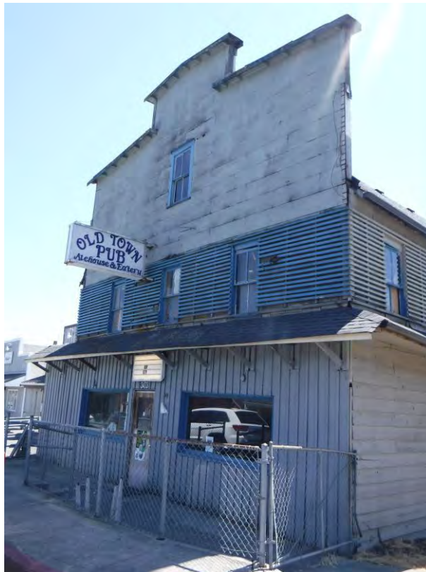
Photograph 1: Northern exterior of building.
