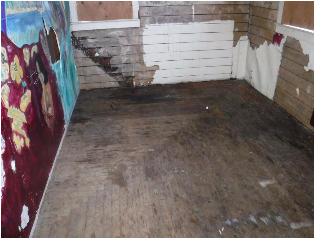
Photograph 11: Typical floor and walls (second floor shown).
