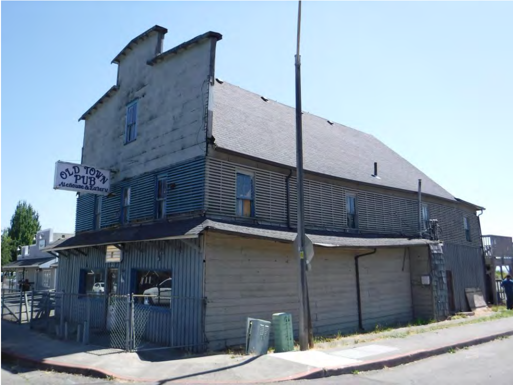
Photograph 2: Northwestern exterior corner of building.
