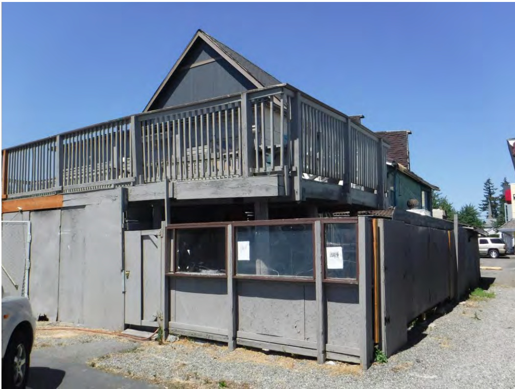
Photograph 5: Deck at southeastern exterior corner of building.
