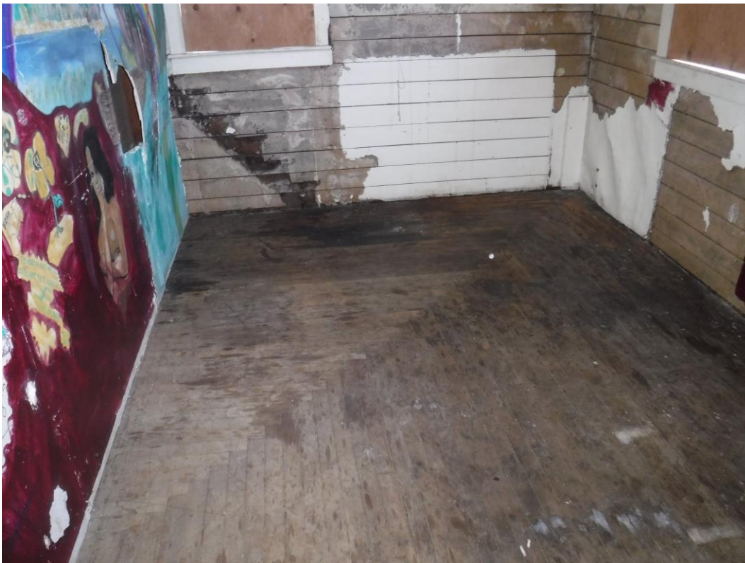
Photograph 11: Typical floor and walls (second floor shown).
