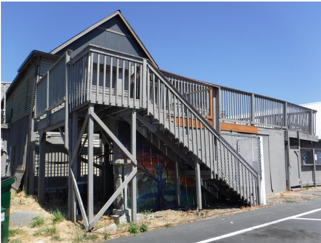
Photograph 4: Deck at southern exterior of building.
