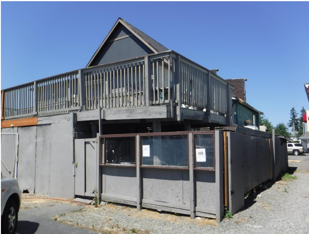
Photograph 5: Deck at southeastern exterior corner of building.
