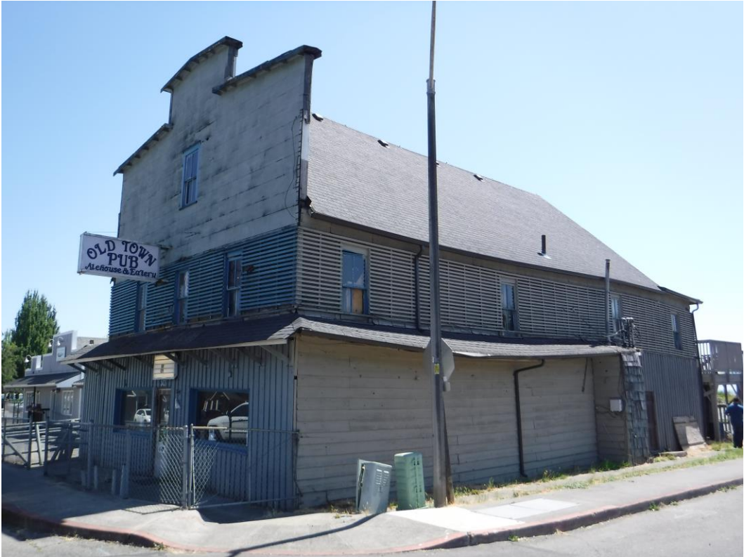
Photograph 2: Northwestern exterior corner of building.
