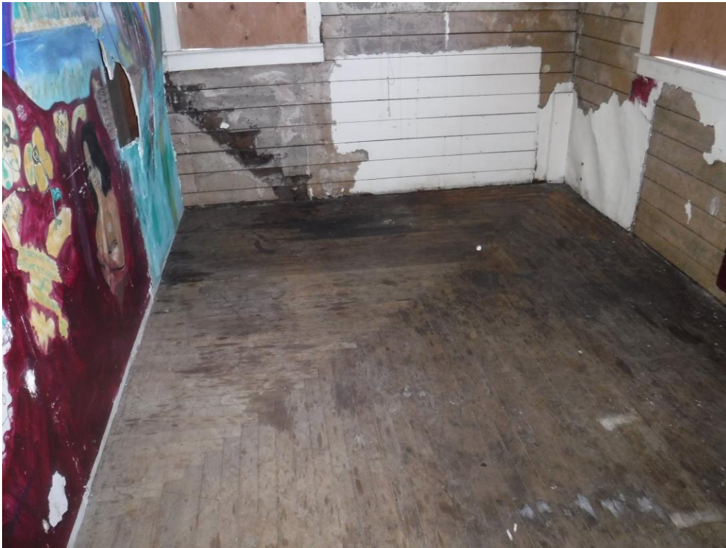
Photograph 11: Typical floor and walls (second floor shown).
