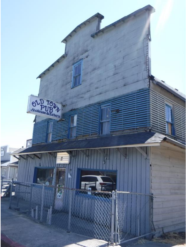
Photograph 1: Northern exterior of building.
