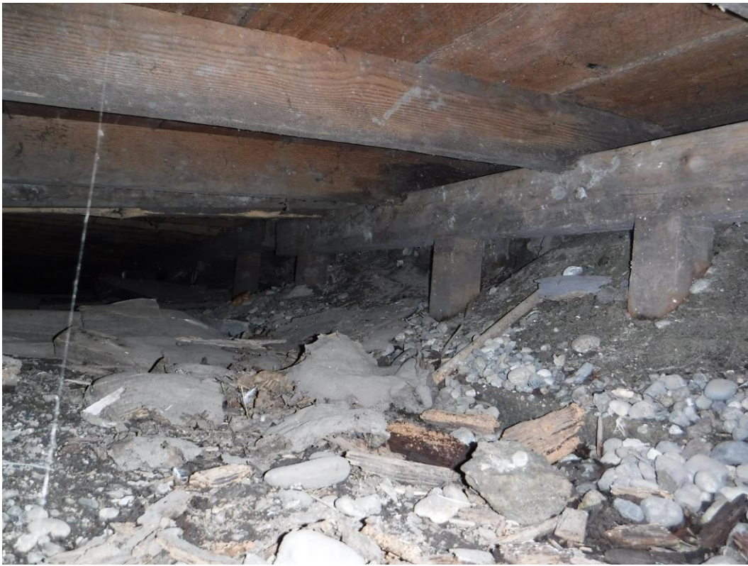
Photograph 16: Typical foundation system and underside of first floor.
