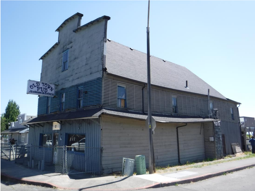
Photograph 2: Northwestern exterior corner of building.
