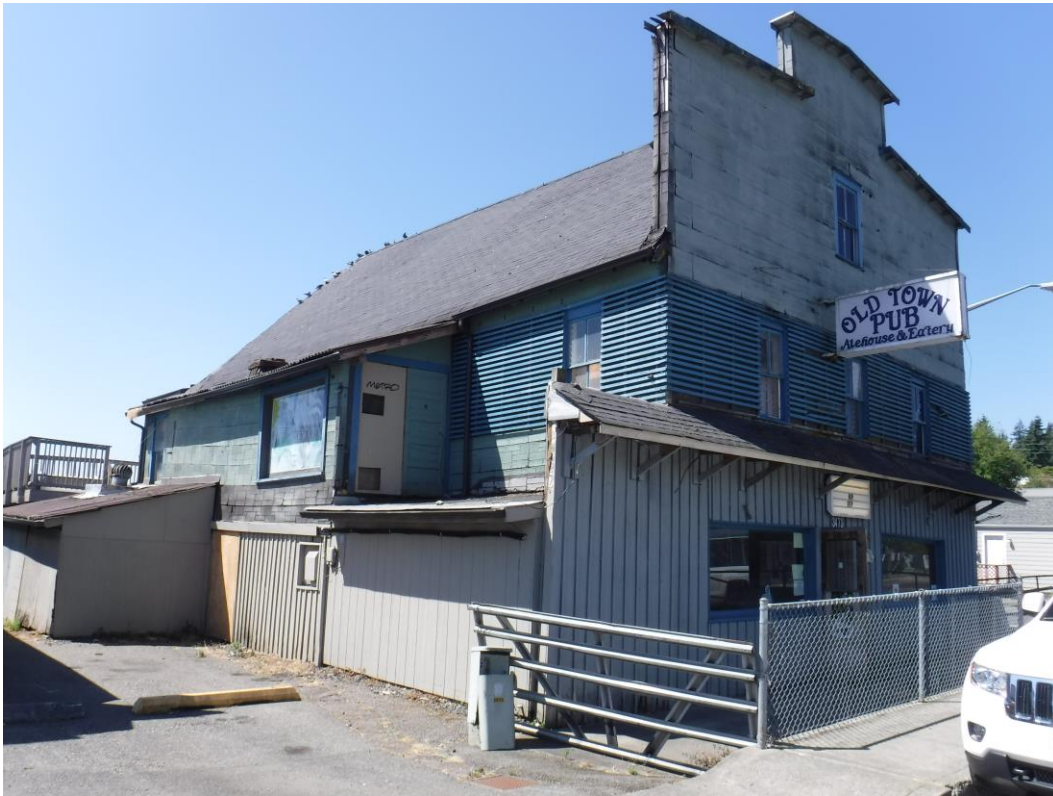
Photograph 6: Northeastern exterior corner of building.
