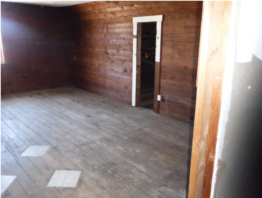
Photograph 13: Typical floor and walls (third floor shown).
