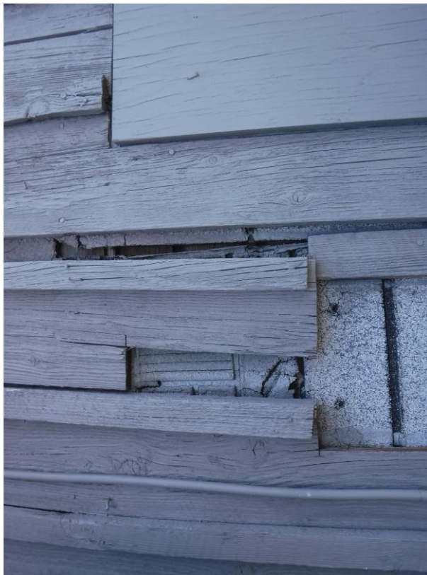
Photograph 7: Typical exterior shiplap.
