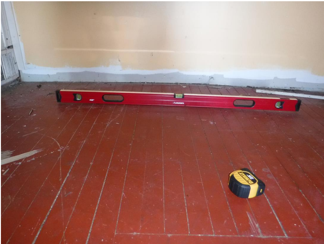
Photograph 12: Second floor at building center with high point (slope east and west).
