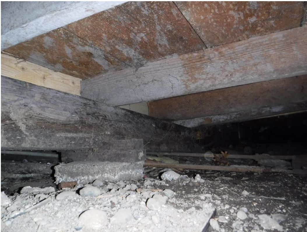
Photograph 15: Underside of first floor.
