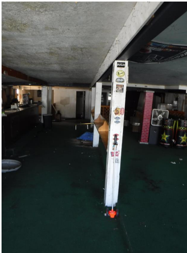
Photograph 9: Interior line of columns at first floor.
