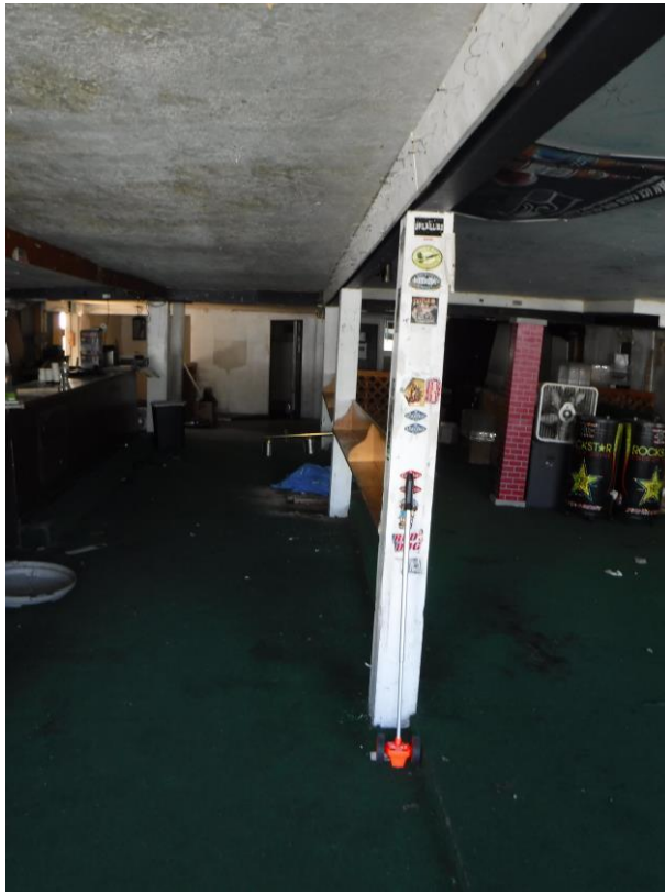
Photograph 9: Interior line of columns at first floor.
