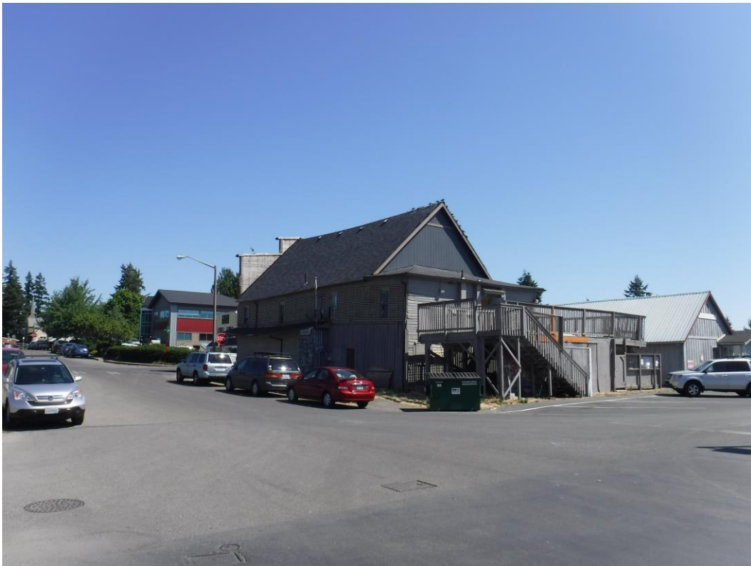
Photograph 3: Southwestern exterior corner of building.
