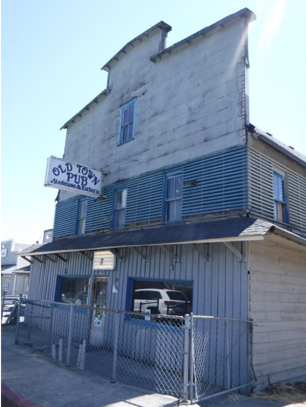
Photograph 1: Northern exterior of building.
